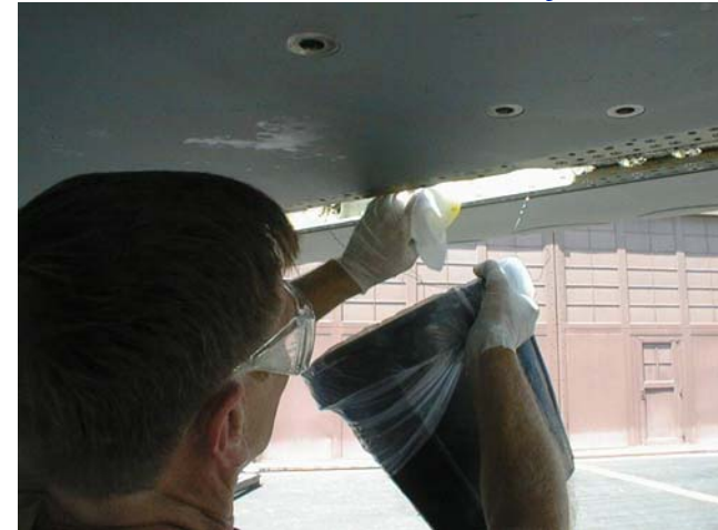
Chromic acid etching process on underwing repair
