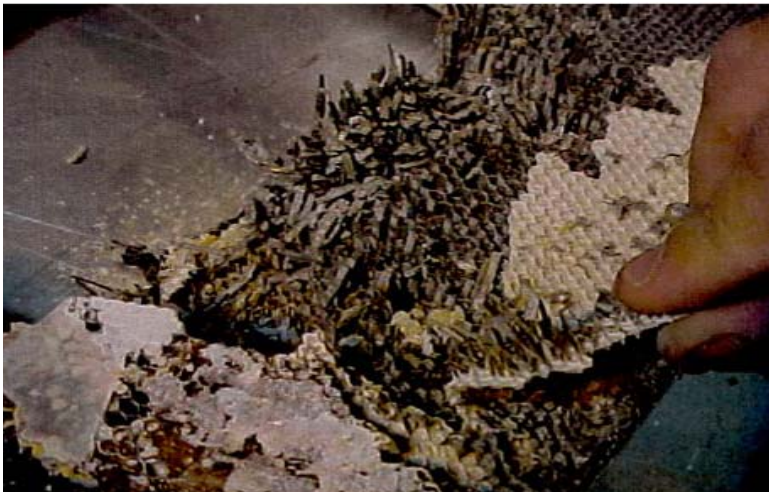
Really corroded core
